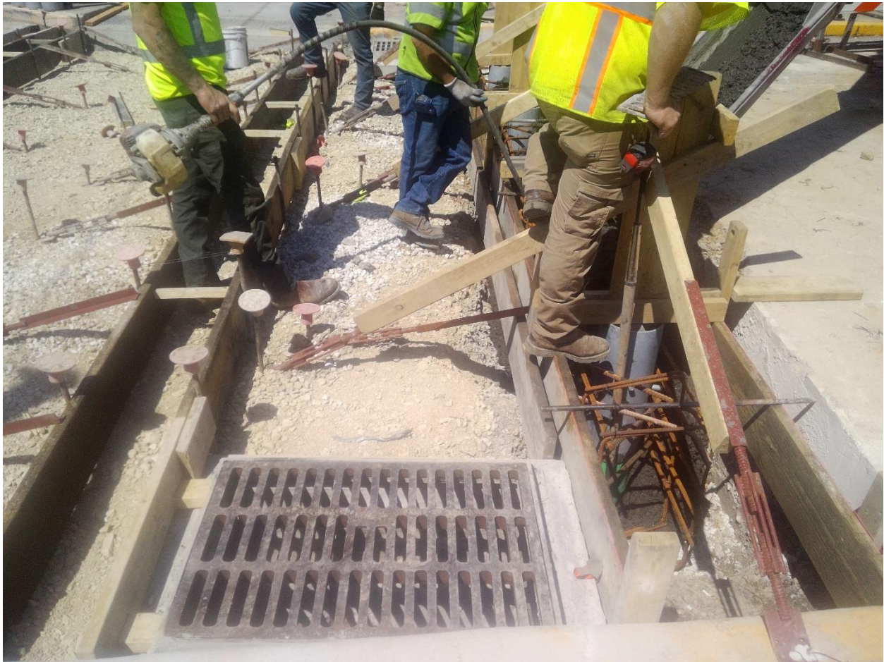
Bollard footer pour at North Washington St., adjacent to the structures/castings that CBU installed for us in a quick timely manner so we could proceed with the project at this location.
